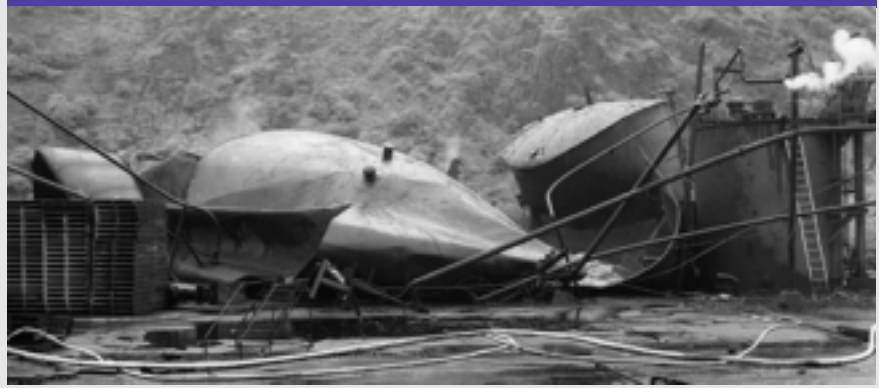
● Figure 8. WESTVACO paper mill tank failure.
